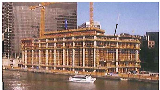
Fig. 6: As of May 2006, construction had progressed to the fourth parking level. The 6 ft (1800 mm) diameter exterior columns signal the scale of the structure to follow
