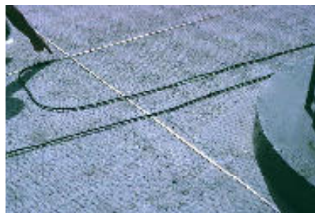
Figure 13 – Cathodic Protection below Mat
