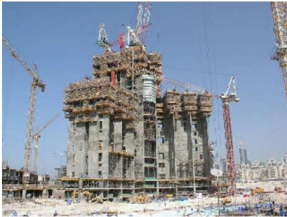
Figure 23 – Self-Climbing Formwork System
